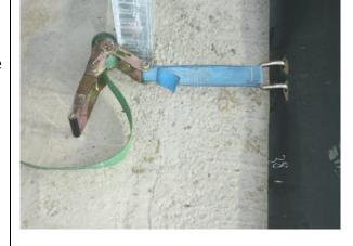
**2)** Using the flat PVC strip and nailins, attach the topcover every foot at the front of the stall.
