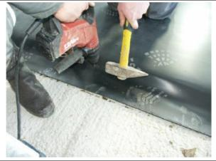
**3)** Fix the topcover with the PVC strips on the front of the stall and at each length following the attachment diagram page 1.
